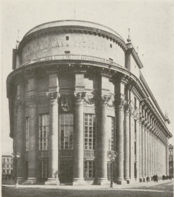
The P. K. O. Building in Krakow.
