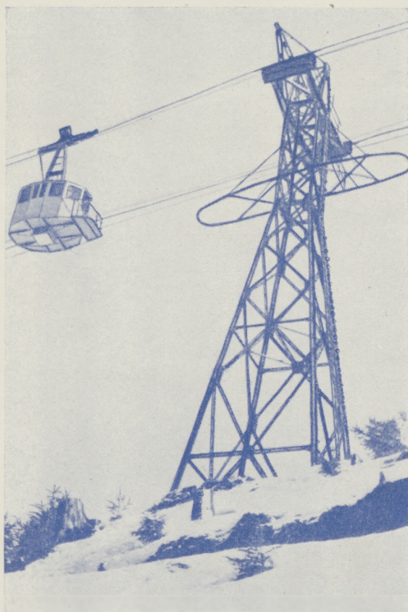
New aerial railway in operation
