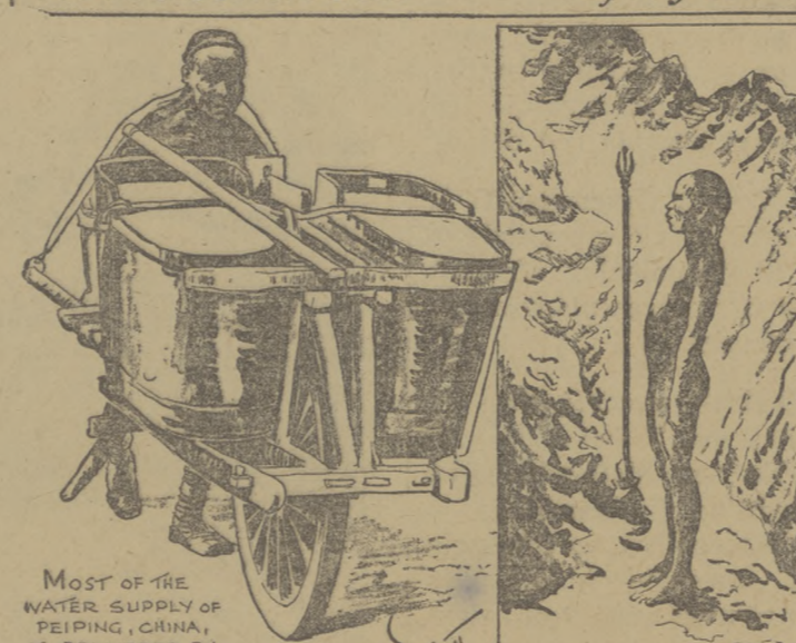
MOST OF THE WATER SUPPLY OF PEIPING, CHINA, IS DELIVERED BY WHEELBARROWS THROUGH THE STREETS OF THE CITY. TIBETAN MYSTICS AFTER YEARS OF TRAINING LIVE NAKED IN THE HIGH HIMALAYAS IN A TEMPERATURE FAR BELOW FREEZING THROUGH THEIR POWER TO GENERATE "GUMO, OR BODY HEAT." THE PERFUMES OF THE FRUIT-FLOWERS AND LEAVES OF THE ORANGE-TREE ARE ALL DIFFERENT.
